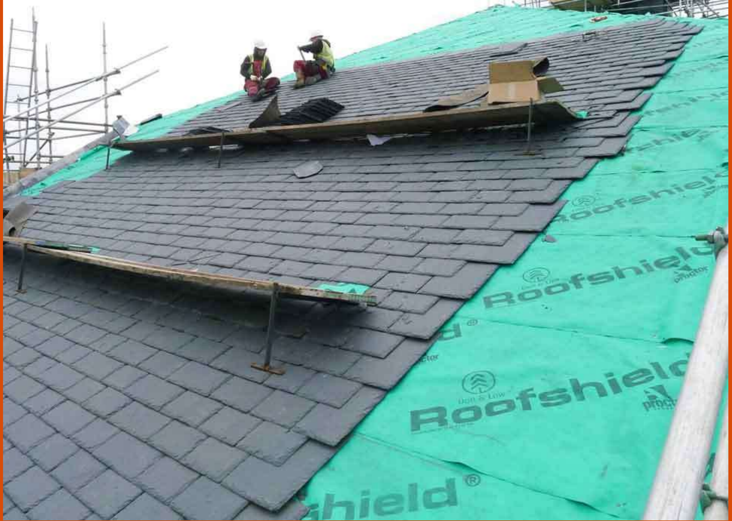
New slate roof – larger slates at bottom, smaller slates at top
