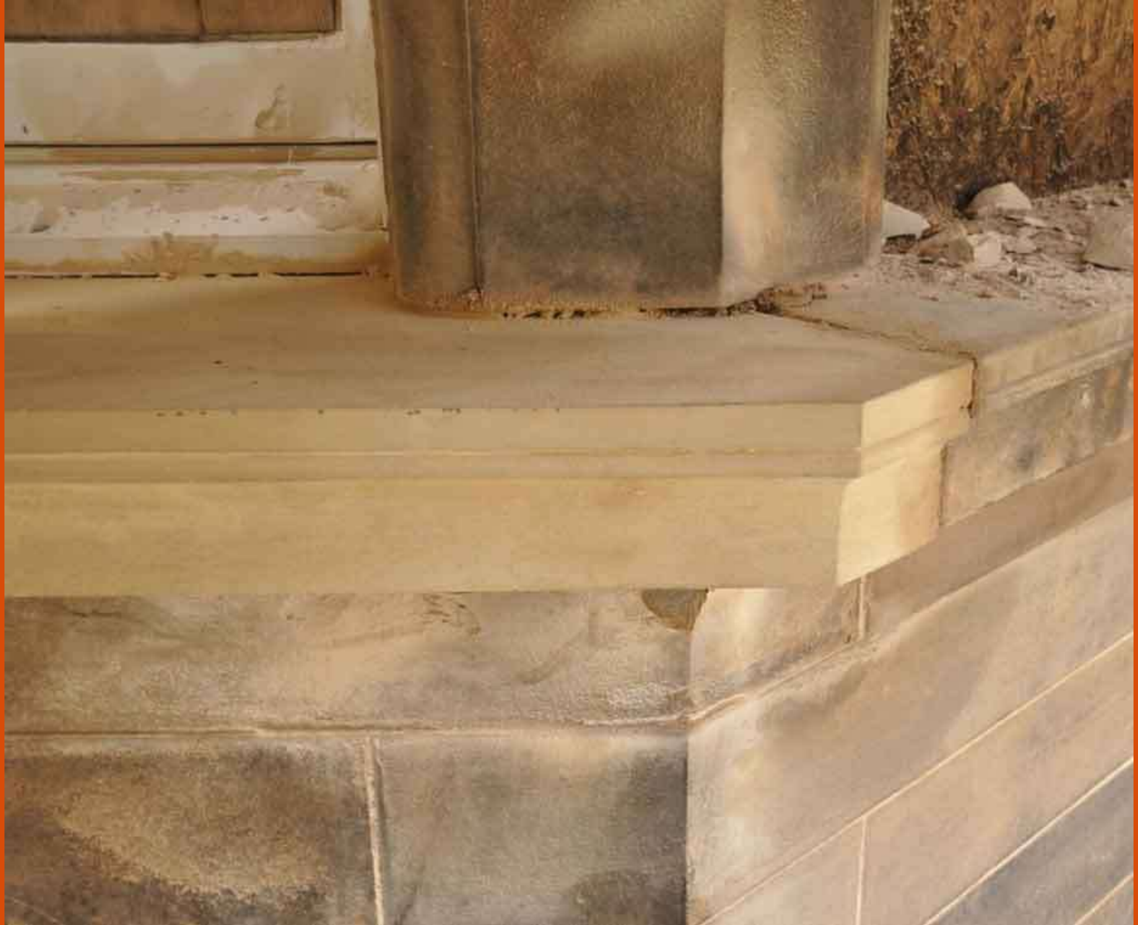
External wall repairs - new stone cill
