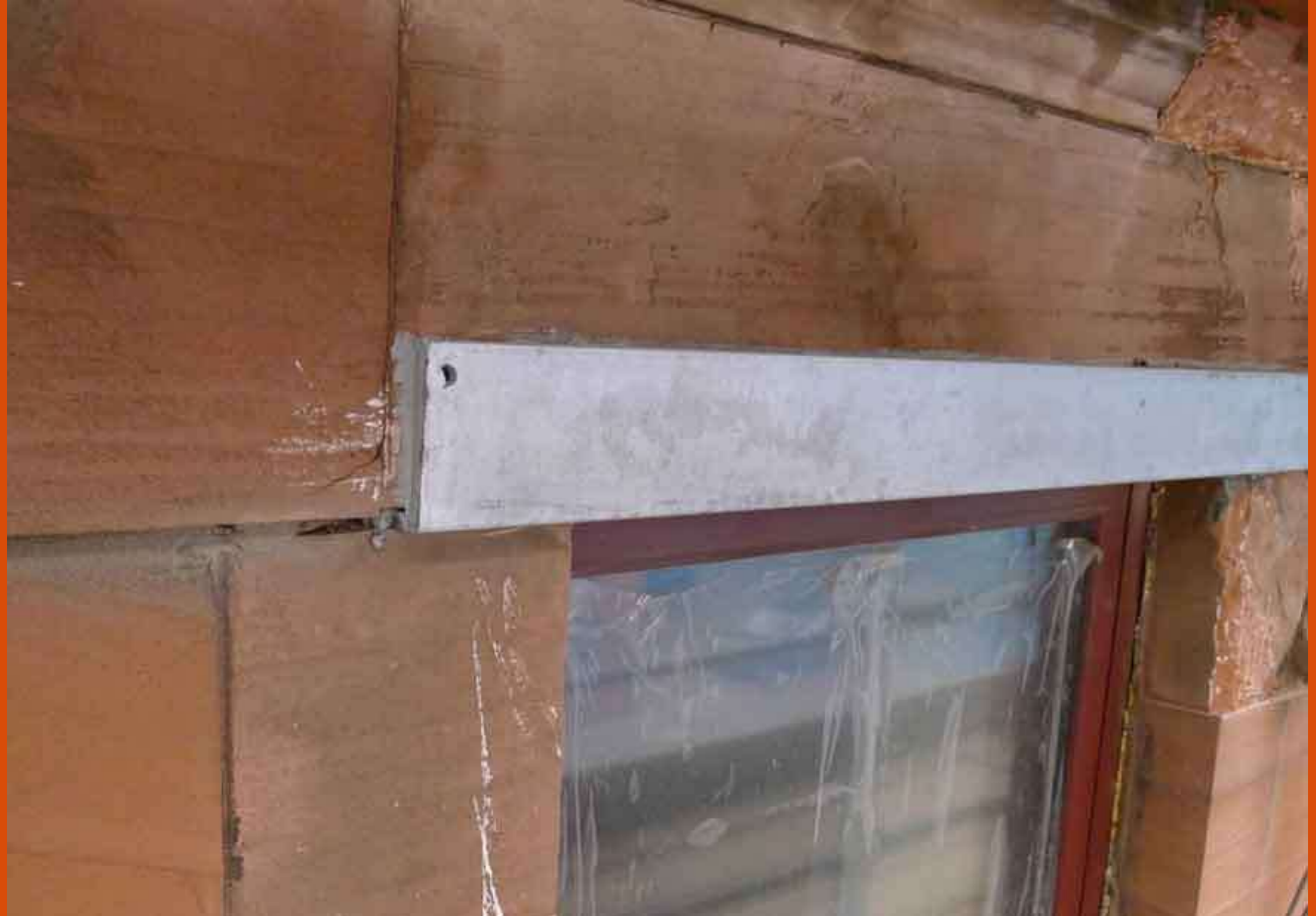
Steel angle lintol repair
