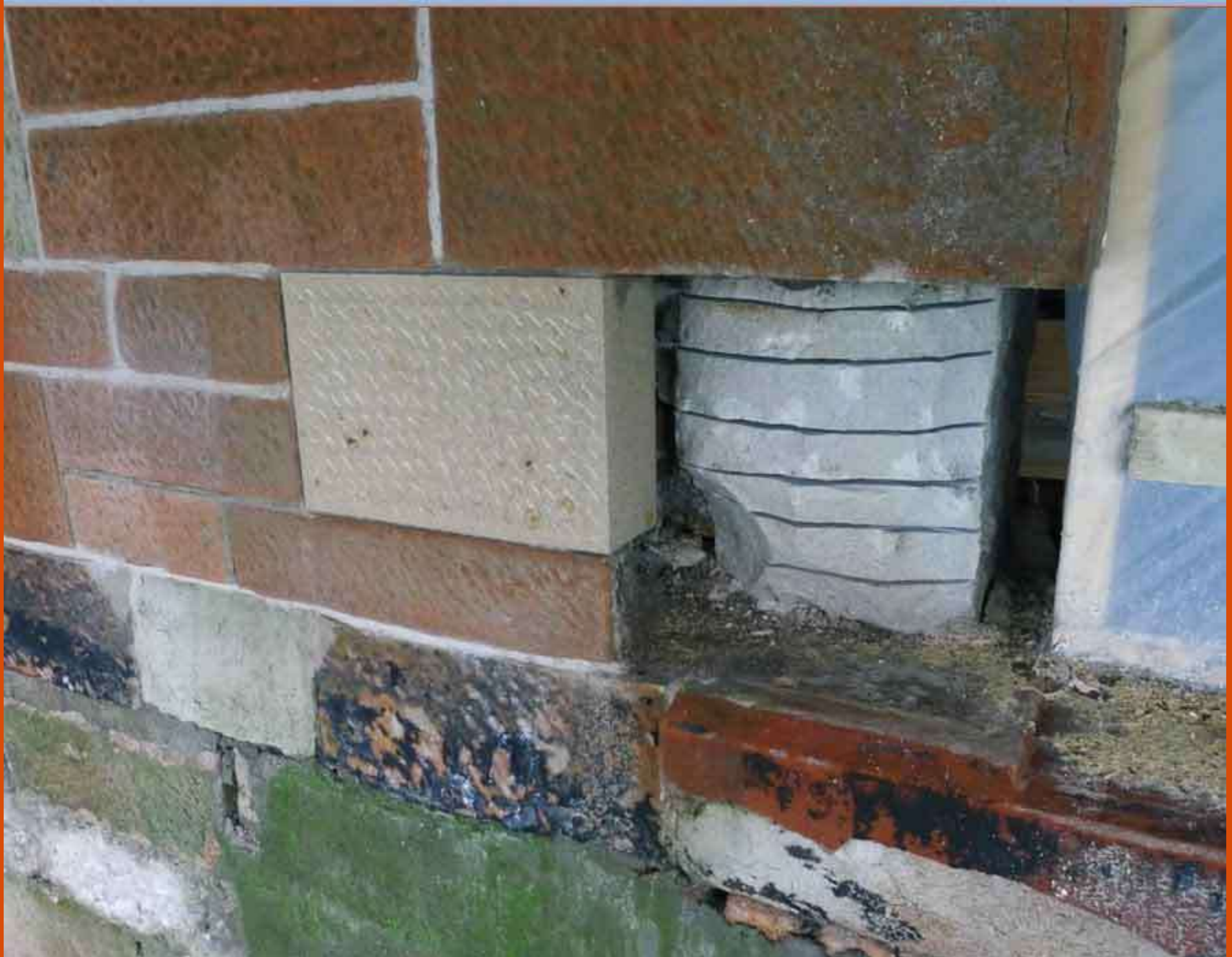
External wall repairs - indenting stone
