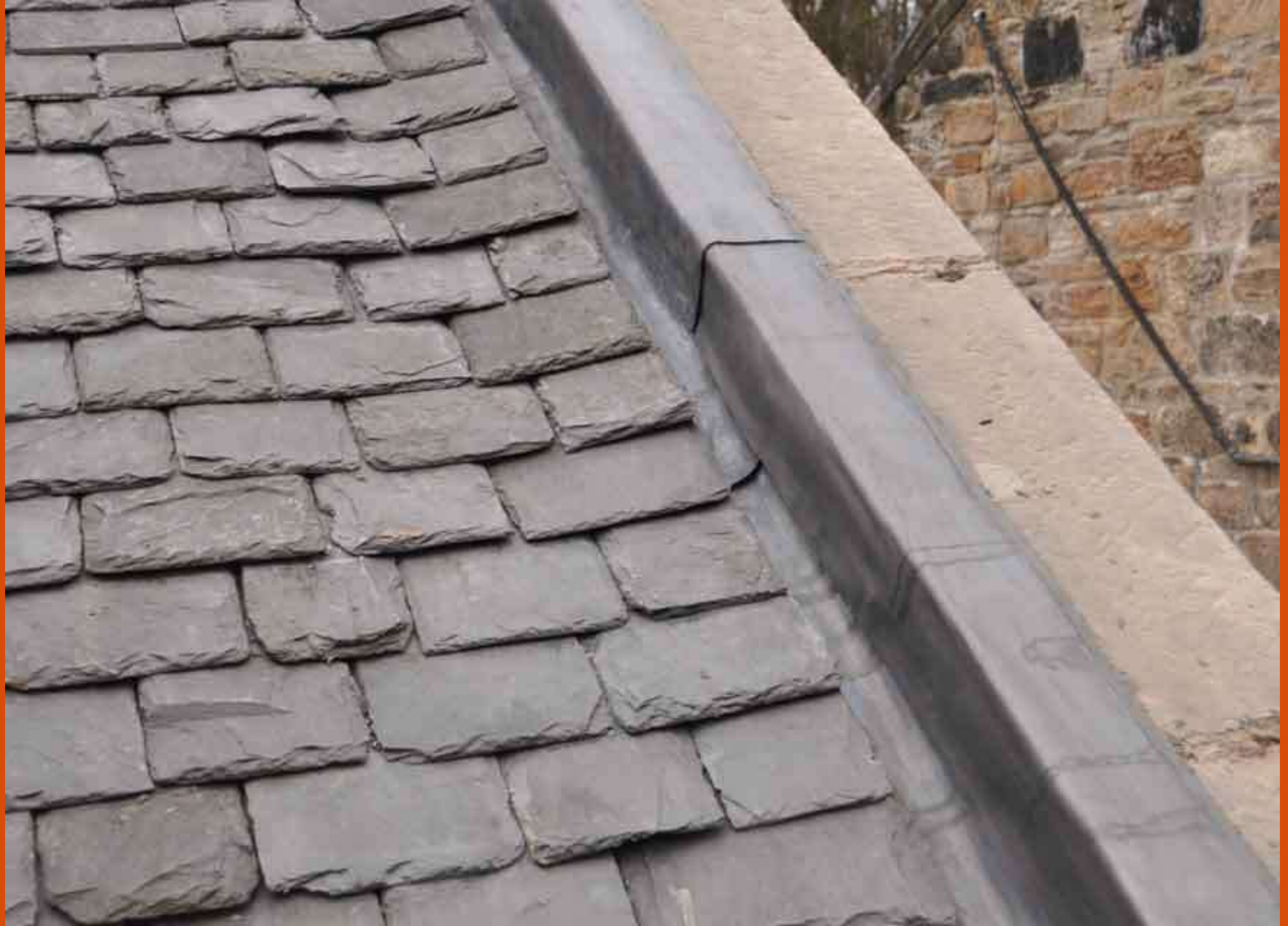
Flashing: skew partially covered in lead
