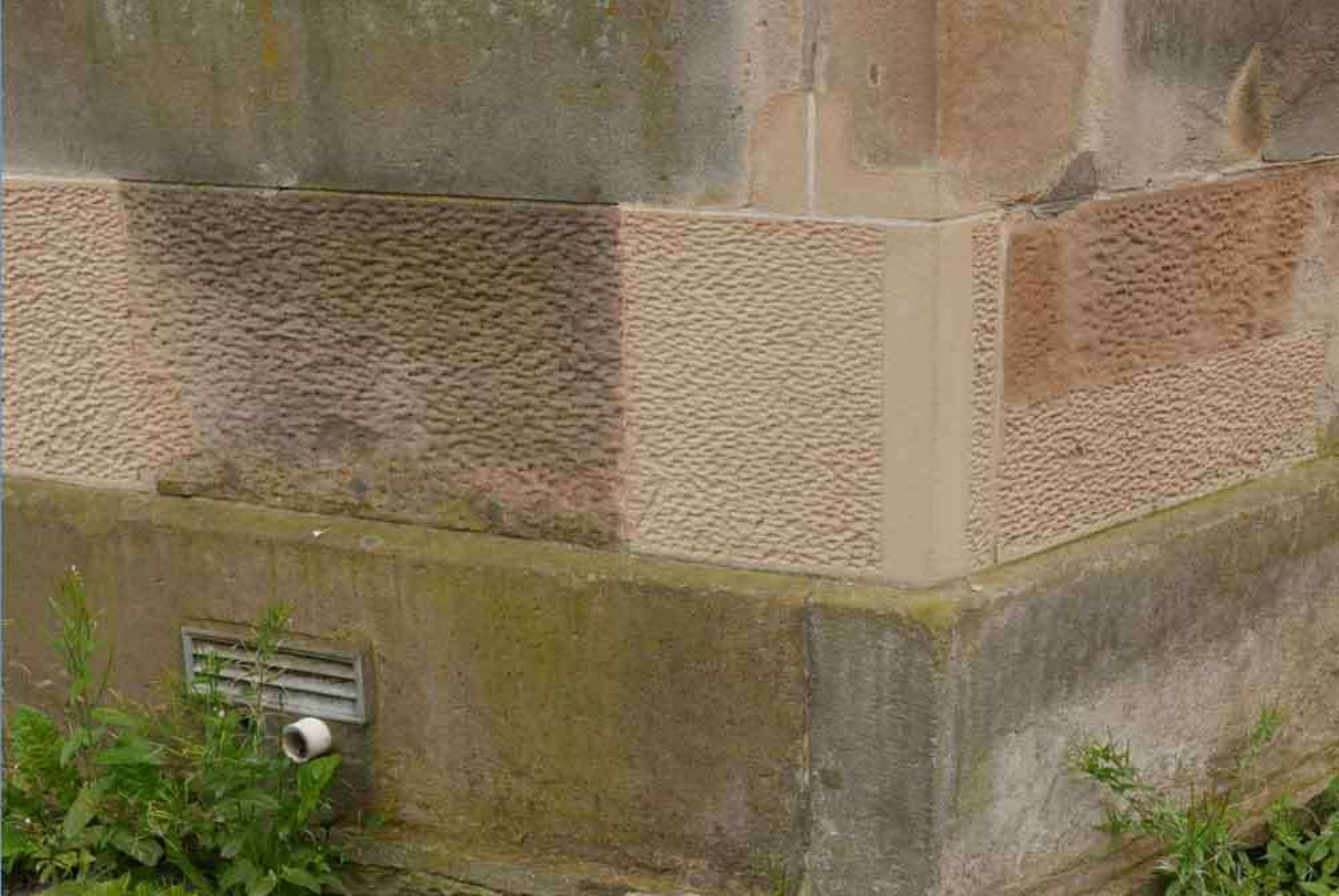
External wall repairs – lime based Lithomex ‘plastic’ repair
