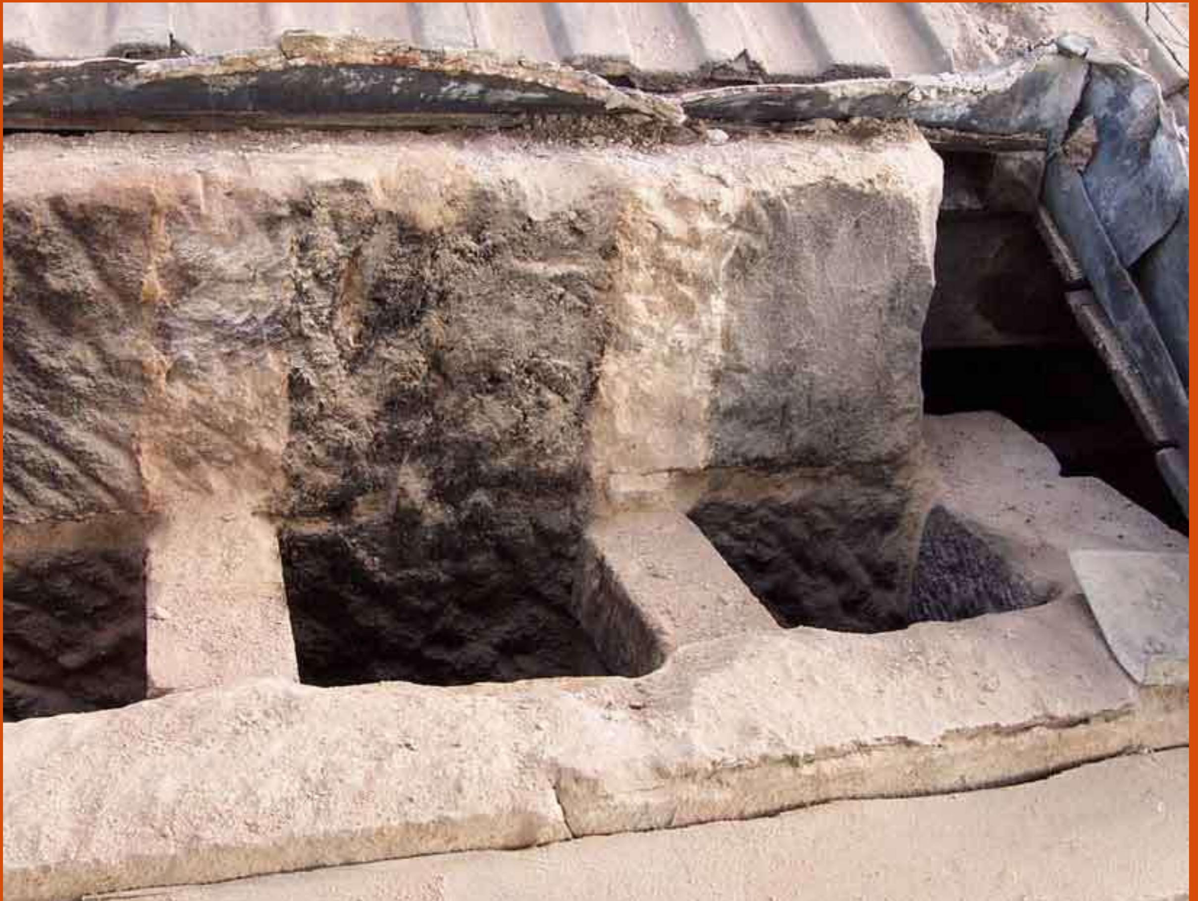
Chimneys - Individual flues are kept separate by bridges
